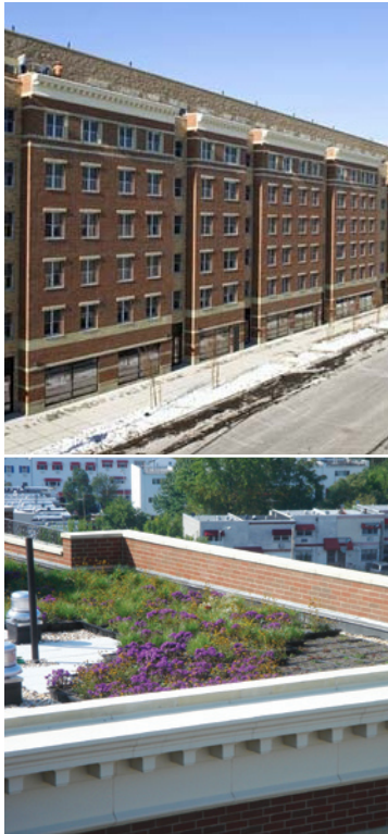
ABOVE Intervale Green offers healthy, beautiful, low-cost rental homes to approximately 400 people, one-third of whom move in directly from homeless shelters. It is the largest affordable, multifamily high-rise building in the United States that is Energy Star-certified, and meets the Enterprise Green Communities Criteria.
