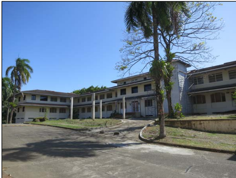
Casa Providencia, the special needs orphanage in Colón, under renovation
